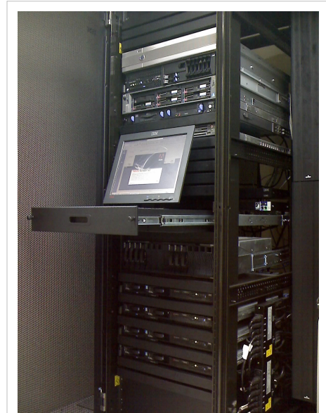
A typical server rack, commonly seen in colocation
