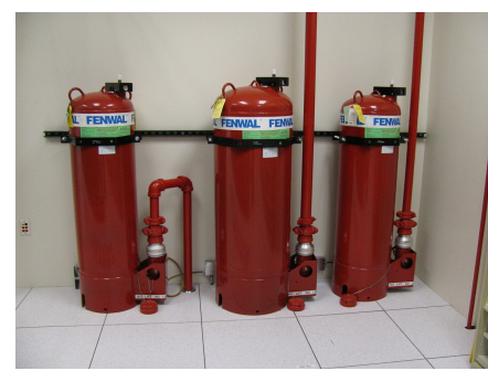
FM200 Fire Suppression Tanks
